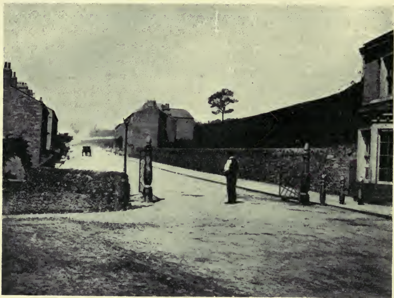
Fig. 85.—TOLL BAR ON WAKEFIELD ROAD, SOWERBY BRIDGE (1824-1870).
