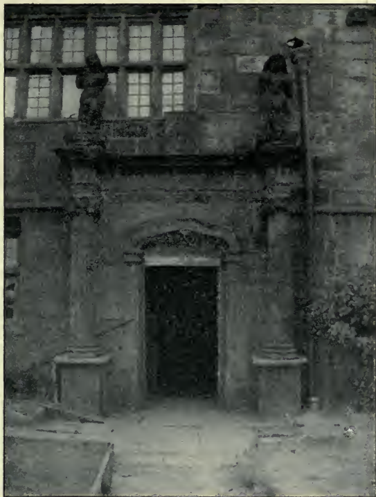
Fig. 43.—HIGH SUNDERLAND, SOUTH PORCH. Photo. H. P. Kendall.
