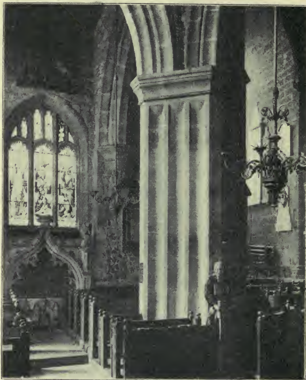
Fig. 24.—LARGE PIER, DESIGNED TO SUPPORT THE EARLIER TOWER.
