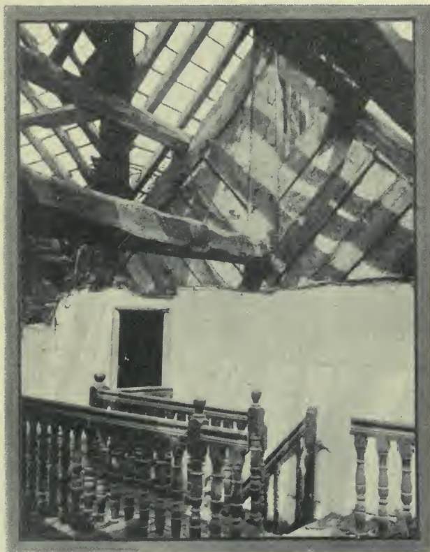
Fig. 21.—TIMBER WORK AT BINROYD.
