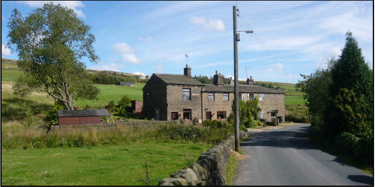
Figure 44. Lumb Terrace, number 1 to number 3 - viewed from the north-west. (2011)
