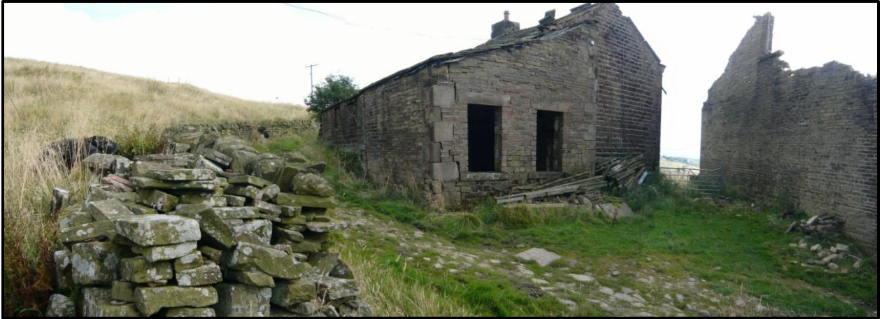
Figure 16. Withins – viewed from the west. (2011)
