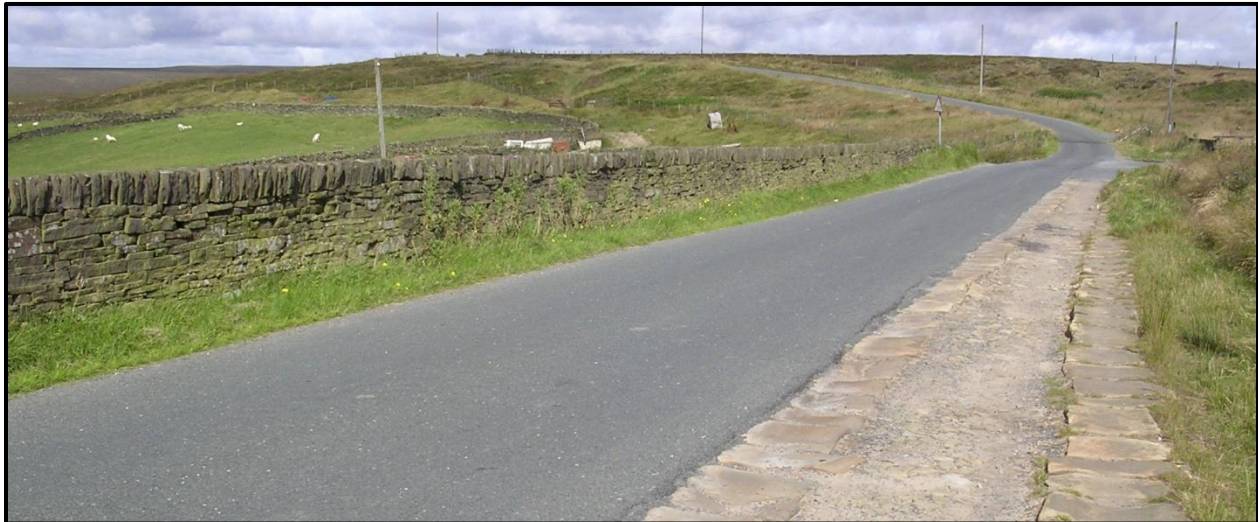
Figure 40. Flagstone road surface laid for the use of horse-drawn carts and wagons on the Cold Edge Road north of the Withins Hotel – viewed from the south. (2010)
