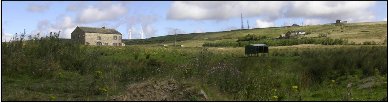
Figure 18. Haigh Cote, now extended, (left) and Withins (right) - viewed from the west. (2011)
